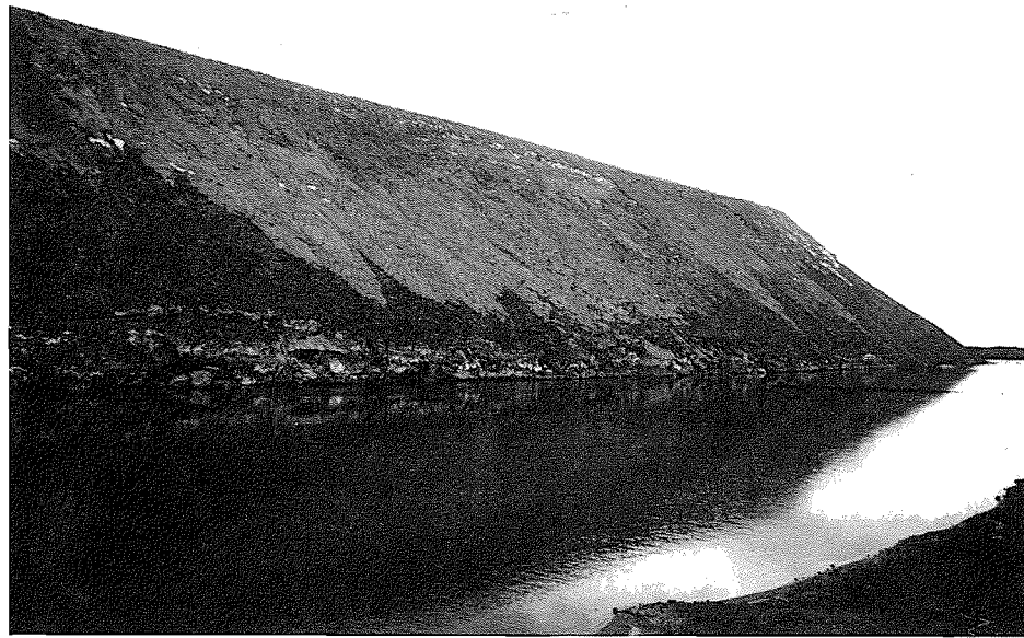
FIG. 1. Tailings pile at the PCS potash mine at Lanigan, Saskatchewan.
