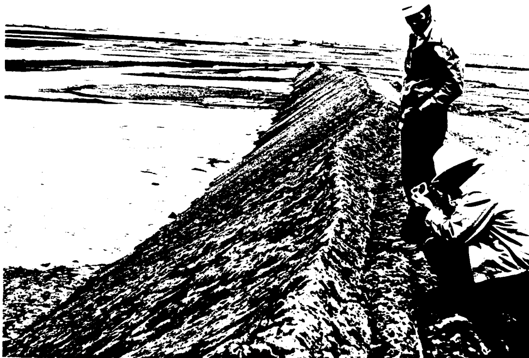
Figure 2 Potash tailings; Angle of repose
